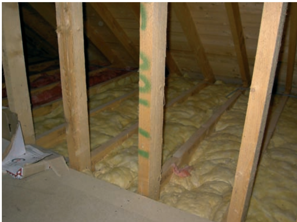
A loft like this one at Spey Bay Hall can top up the roll-out insulation to make it up to 275-300mm
