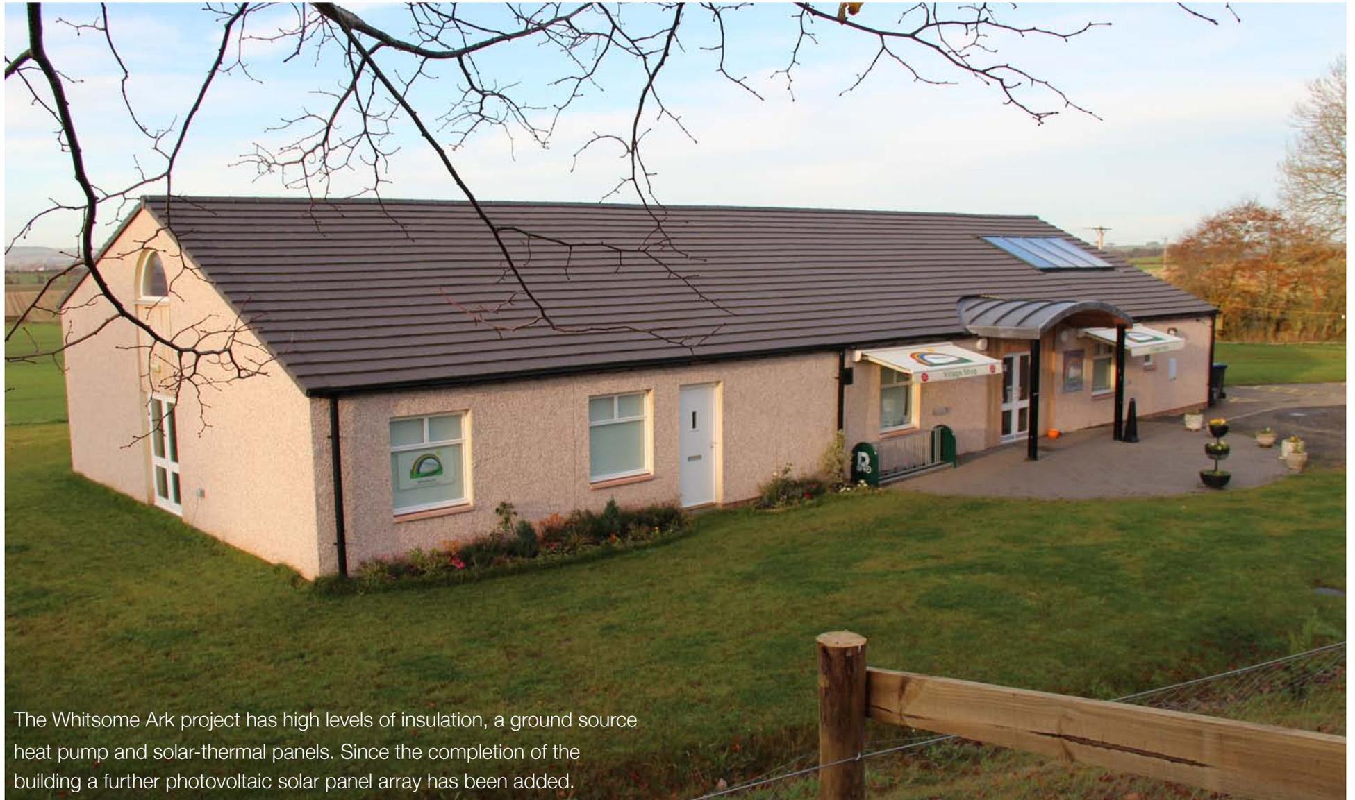
The Whitsome Ark project has high levels of insulation, a ground source heat pump and solar-thermal panels. Since the completion of the building a further photovoltaic solar panel array has been added.
